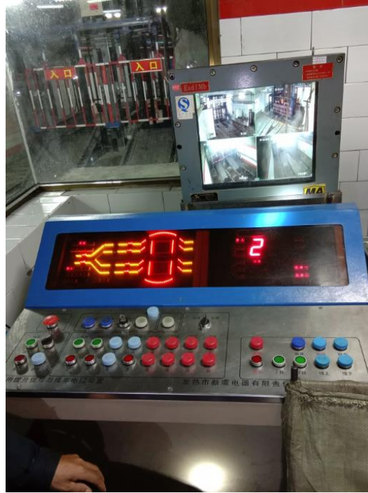
Underground transportation control center
